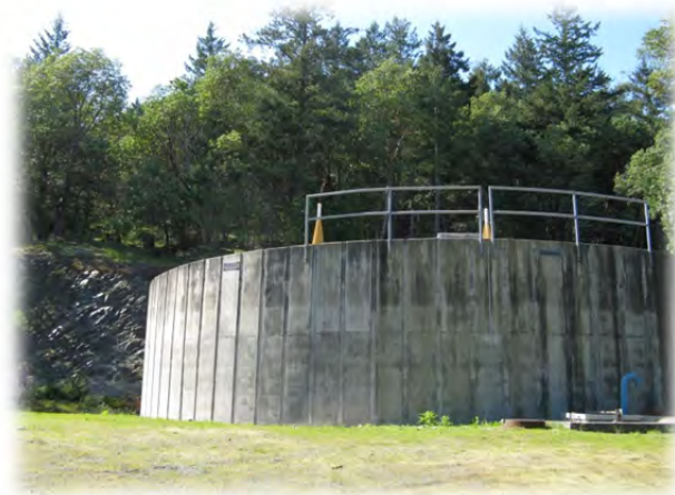
Photo of Fairwinds Reservoir No. 1
