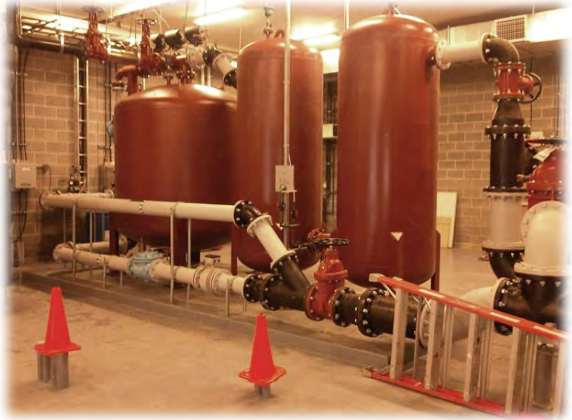
Completed Water Filtration Plant Filtration chambers shown
