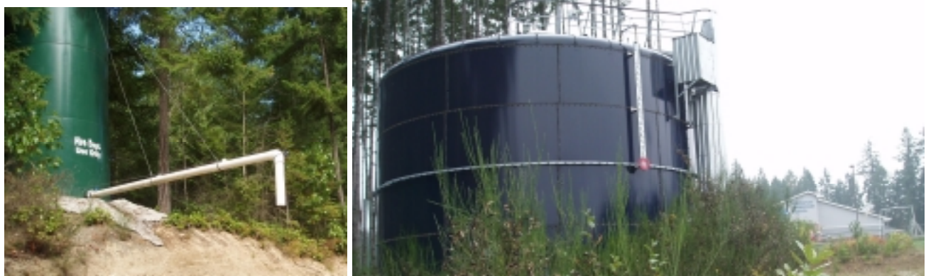
Plates 7 and 8. Errington has achieved Strategic Tanker Shuttle rating by locating permanent, reliable water sources for firefighting throughout the district.
