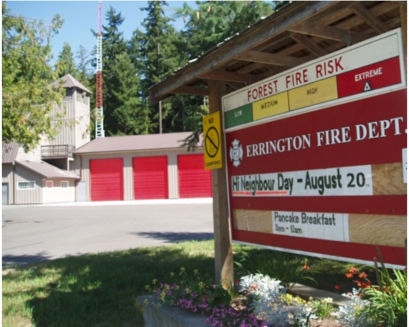
Errington Volunteer Fire Department #1 Firehall
