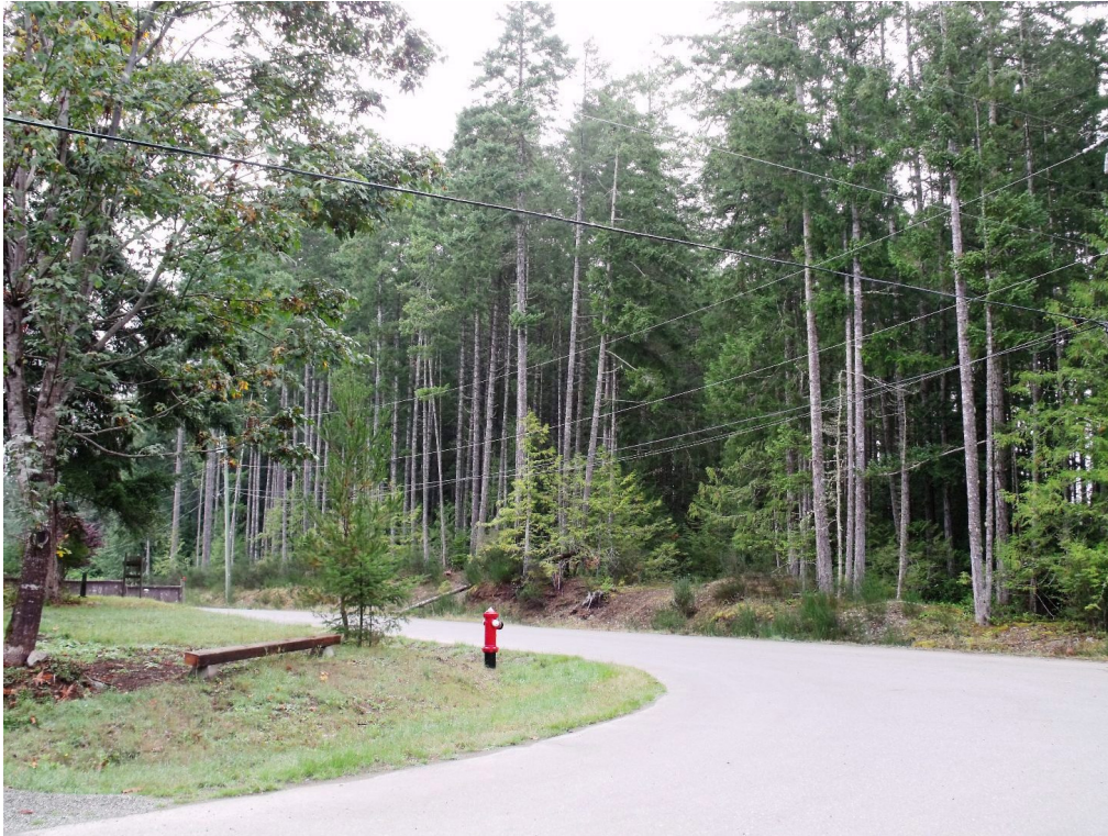
Photo 3 An example of the interface, at the junction of Huckleberry Lane and Dewberry Way.
