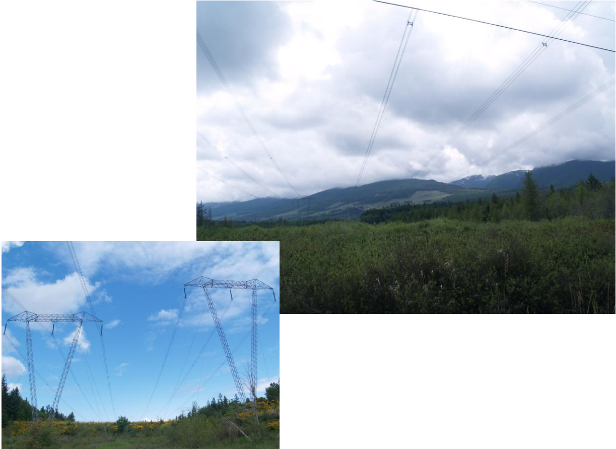
Photos. BC Hydro power transmission line in the area.
