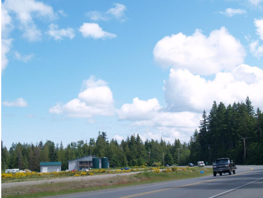
Photo. Highway 4 passes beside Coombs-Hilliers Fire hall No. 2.
