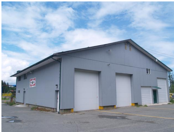
Photo. Fire Hall No. 2.
