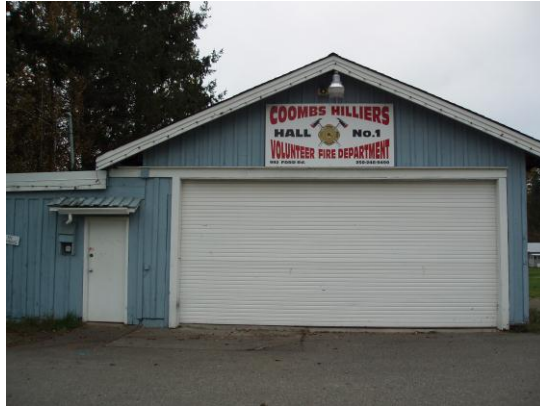
Photo. Fire Hall No. 1.
