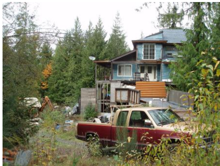
Photo. A number of residential structures at Coombs-Hilliers are not built to building code standards.
