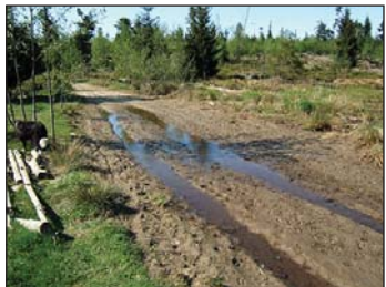
Signs of motorized vehicle use and erosion on trails in the 707CP
