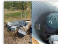
Drilled Wells in Pits
