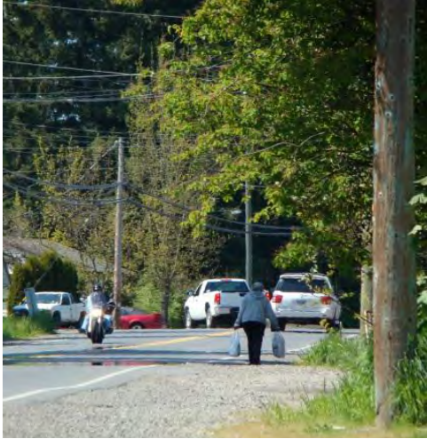
Narrow paved road shoulder is not well suited for cyclists. Uneven and loose terrain is a challenge for pedestrians with reduced mobility.
