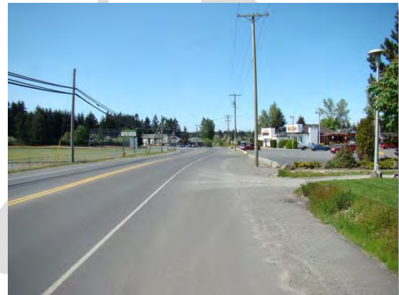
Recent resurfaced section of Cedar Road showing section of widened shoulder near the intersection of Hemer and Cedar Roads.
