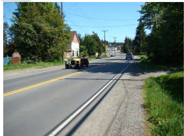
Looking south east along Cedar Road showing lack of paved shoulders and sections of open drainage ditch.
