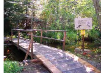
21 Counting Station Bridge
