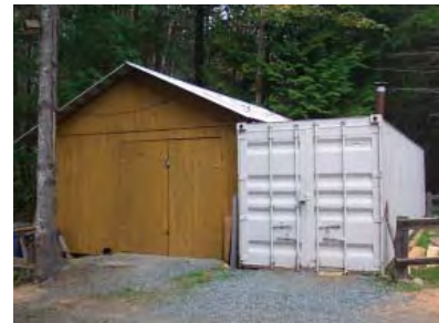
⑨ Hatchery Buildings 1 & 2
