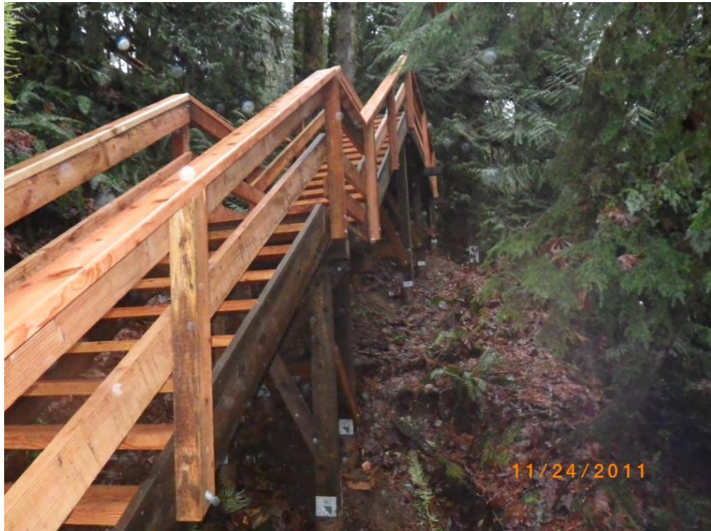
Figure 16. Stairs installed in steep, sensitive terrain within Stocking Creek Regional Park, in the Cowichan Valley Regional District park system.
