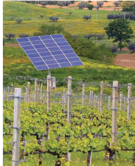
Solar photovoltaic systems can help offset power generation at farms, orchards or wineries.
