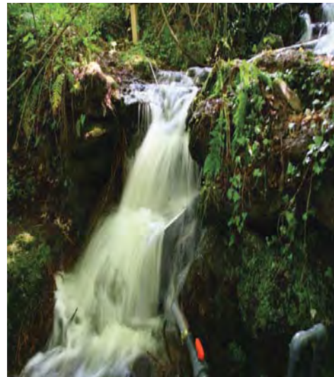
An example of an intake.
