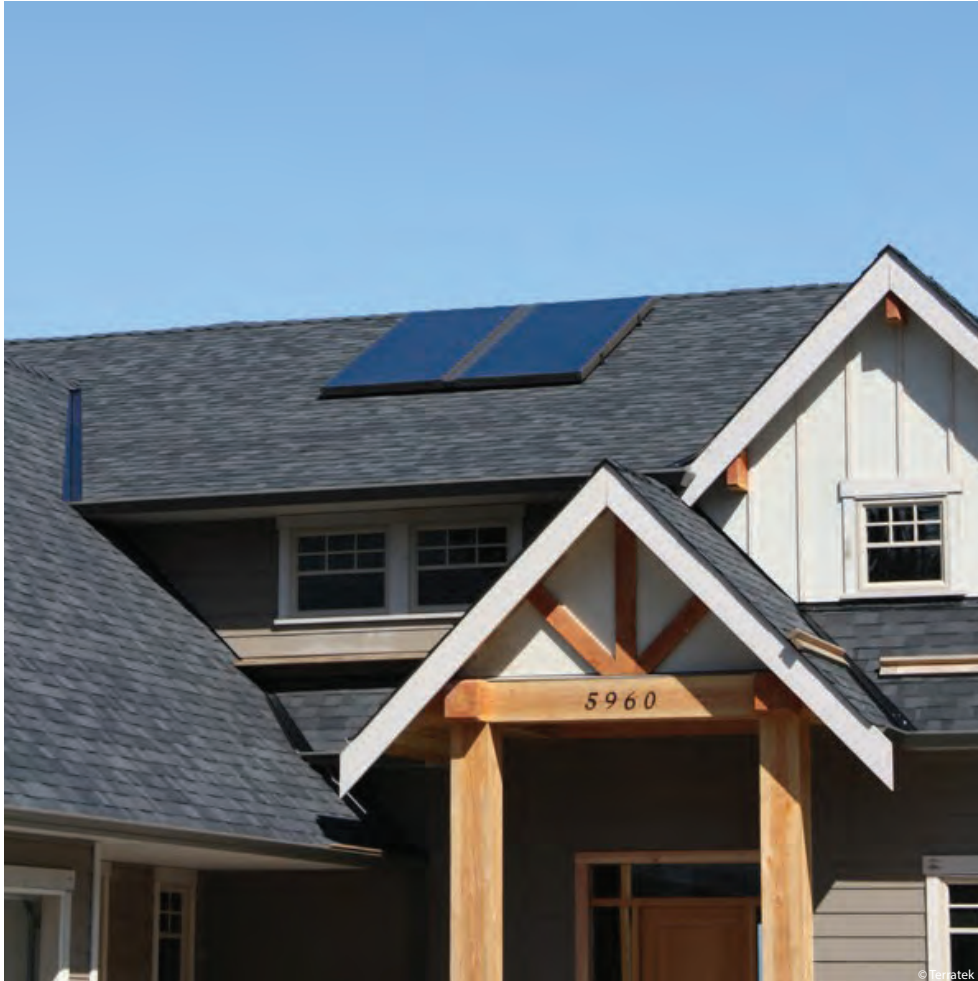
Solar domestic hot water system.
