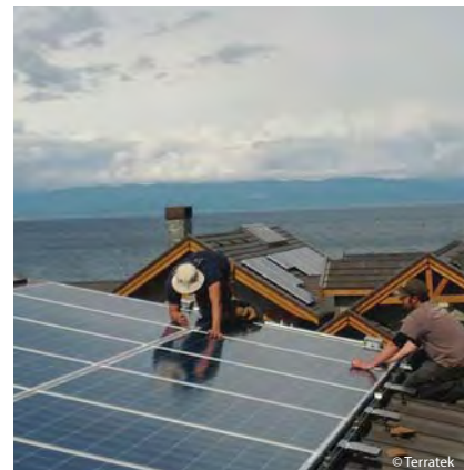
22 kilowatt solar photovoltaic roof installation, Comox, BC.
