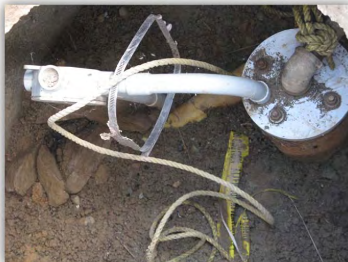
Rollo McClay Wellhead Close-up in 2012
