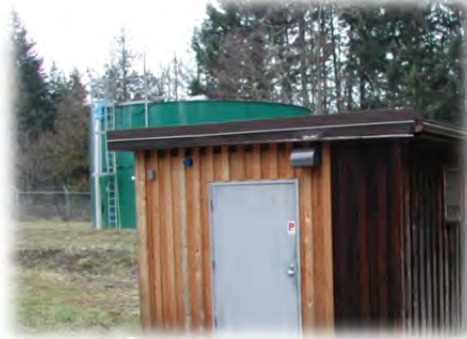
French Creek Main Pumphouse and Reservoir
