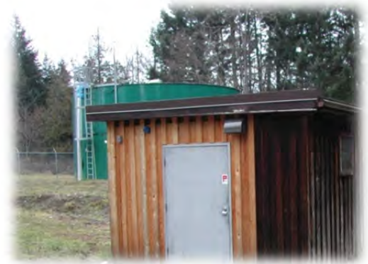
French Creek Main Pump House and Reservoir
