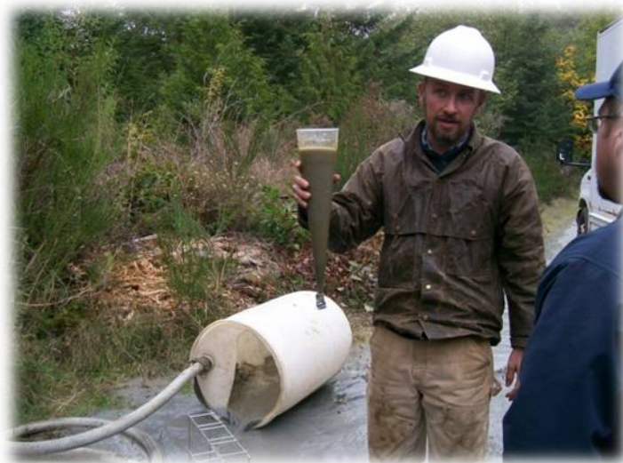
Well Rehabilitation in October 2010
