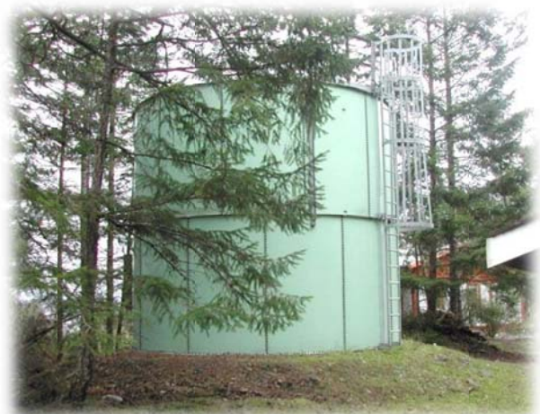
Decourcey Water Storage Reservoir
