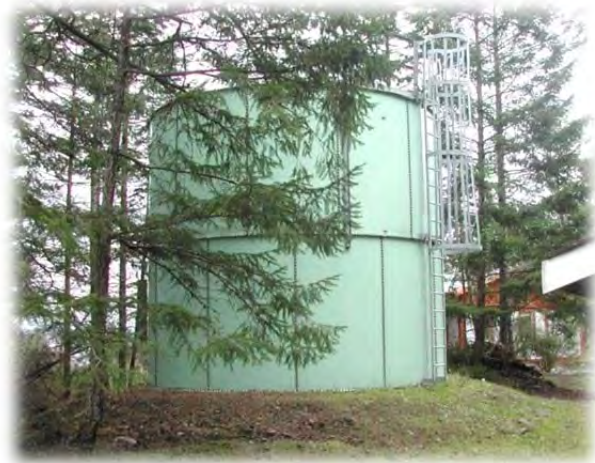
Decourcey Water Storage Reservoir
