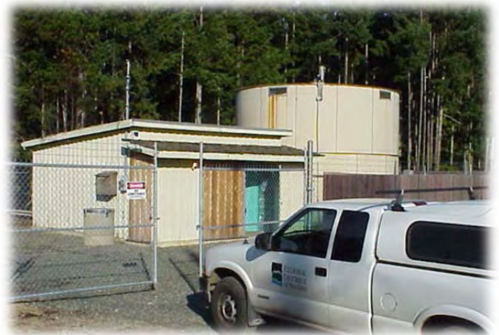
Melrose Pumphouse and Reservoir
