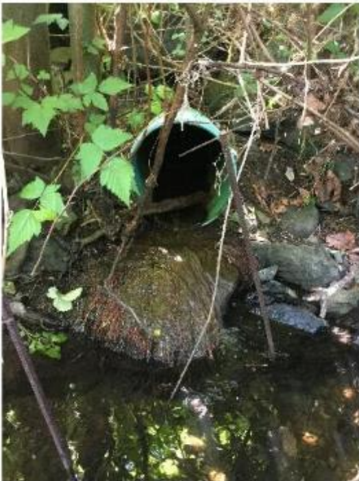
Photo 3) Reach 1, Pool 5 right bank storm pipe outlet
