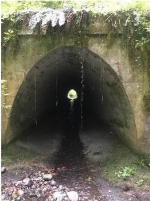
Photo 1) Reach 3 cement culvert under railway track
