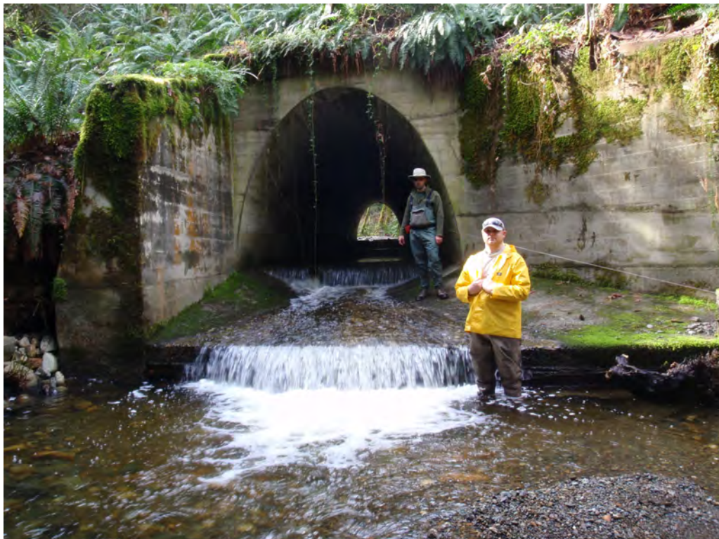
Photo 15. Downstream side of perched Southern Railway culvert crossing in Thames Creek, 4 March 2010.
