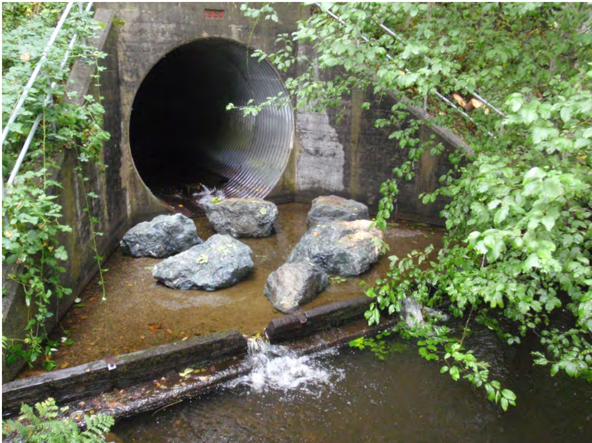
Photo 17. Six over-sized boulders placed on downstream side of Highway 19A culvert in Thames Creek.
