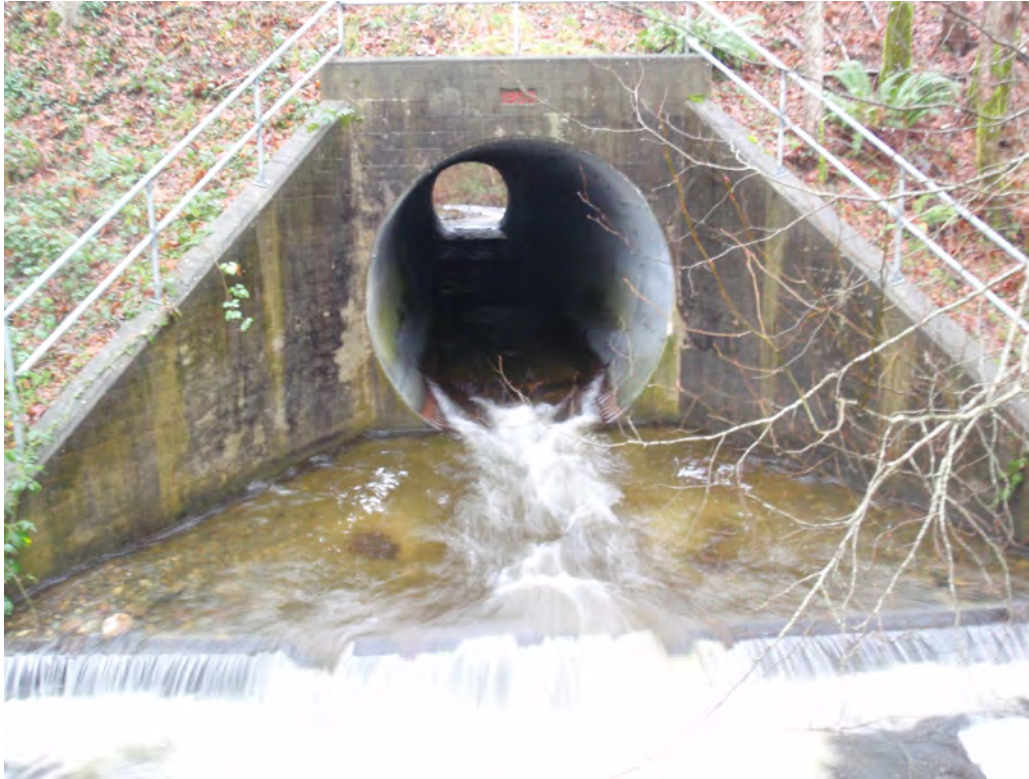
Photo 14. High velocity discharge across concrete apron in Thames Creek at Highway 19A crossing, 14 January 2010.
