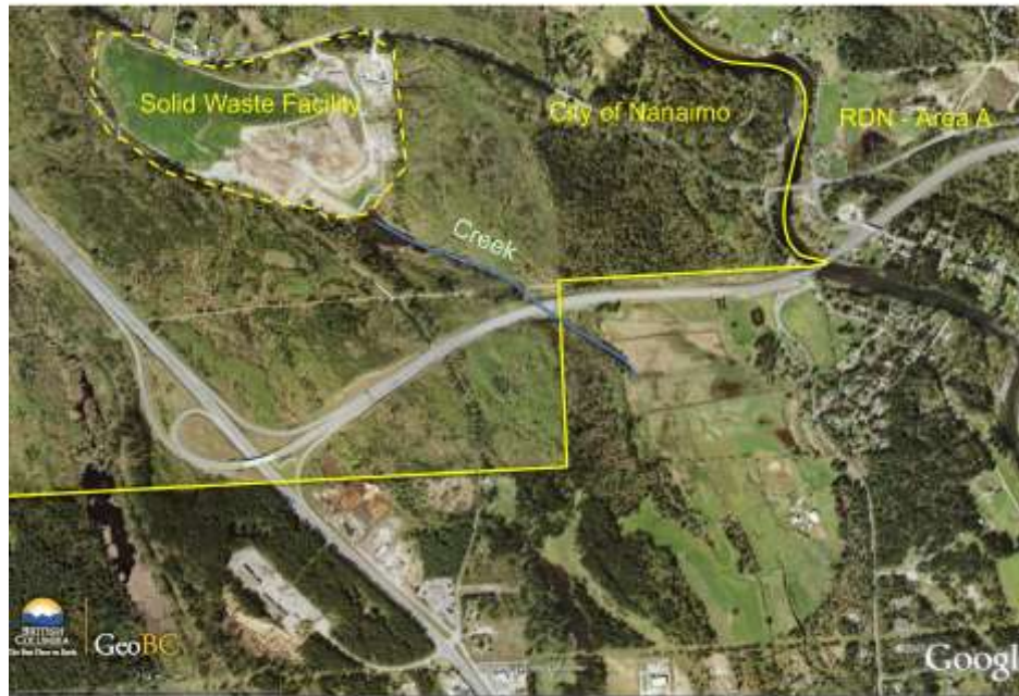
Figure 43: Circle 9 shows the RDN solid waste facility (landfill) in the City of Nanaimo, bordering Area A. Although controlled by a leachate collection system, part of the leachate created by the landfill discharges into a drainage at the southeast corner of the landfill. This drainage flows east, southeast into Area A. Water quality parameters mainly indicate low pH, and the presence of metals (iron, manganese) mostly associated with organic degradation (Morrow 2001).
