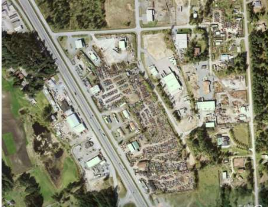
Figure 35: Detail of Circle 1. Potential contaminants associated with auto wrecking and salvage yards will include hydrocarbons, cooling fluids, and metals.
