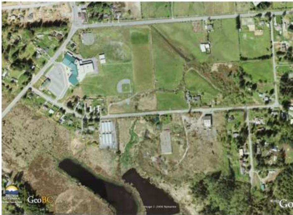
Figure 42: Circle 8 shows a high school and residential lots. The school is now connected to a sanitary sewer however the other properties still discharge their liquid effluents to the ground. Potential contaminants associated with the discharge of liquid waste include bacteriological contaminants (viruses and bacteria), pharmaceutical products and endocrine disruptors (now referred to as Pharmaceutical and Personal Care Products – PPCP)
