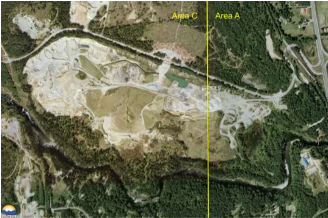
Figure 37: Circle 3 shows gravel pits. In such areas, the dry overburden is removed, thus reducing the filtering effect of the soils above the aquifer(s). Other activities such as asphalt production may take place in gravel pits; potential contaminants include hydrocarbons.
