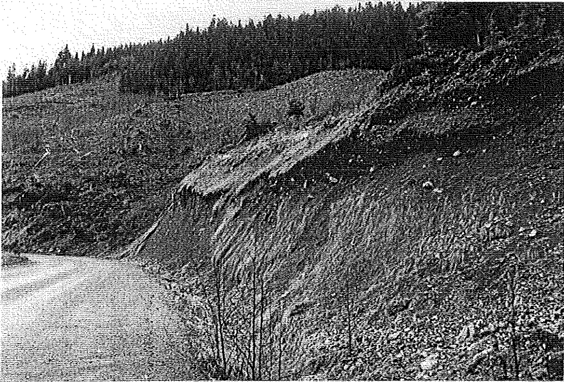
Plate 32. Deep silt till in road cuts near Yellow Creek crossing.
