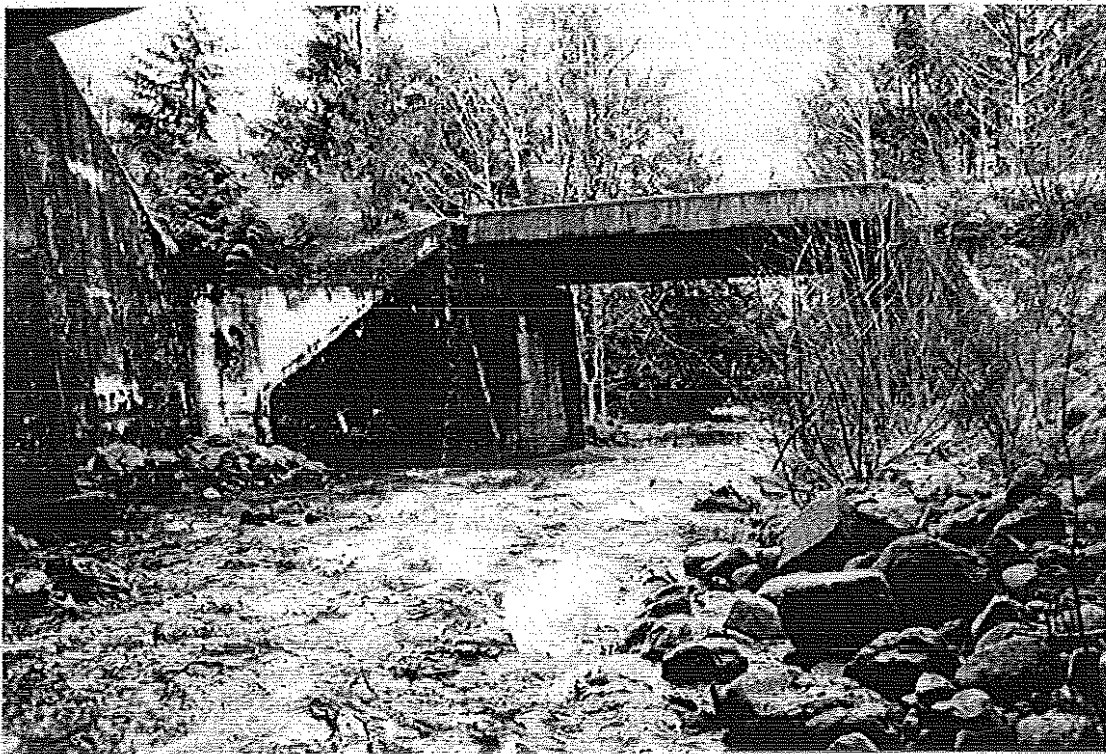
Plate 2. Stop #1. Looking downstream at Lockwood Creek from highway bridge toward railway bridge.
