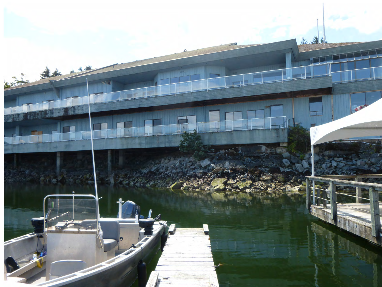
EXISTING SITE PICTURES
