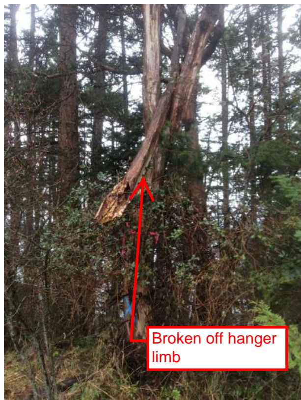
Figure 6: Photo showing Urgent Removal –Tree #1 (Arbutus) at parking lot
