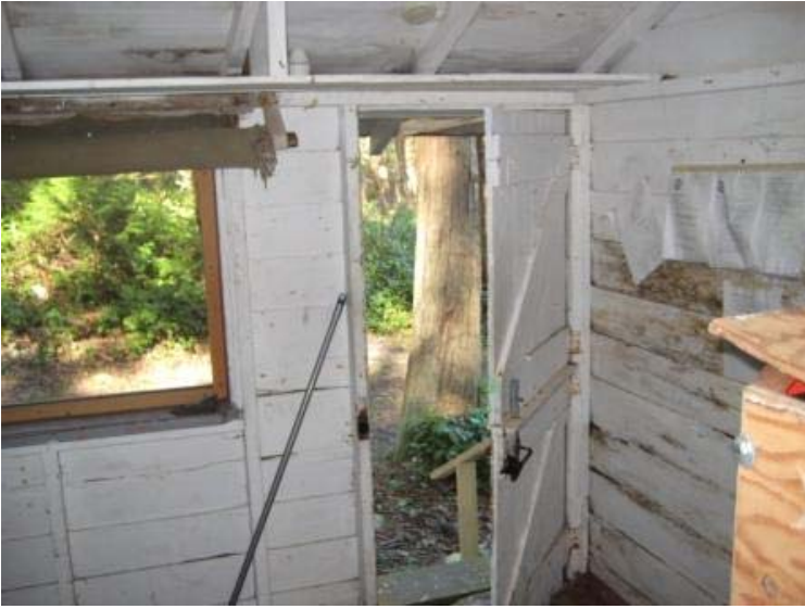
Interior views of one of the older cabins (typical interior)
