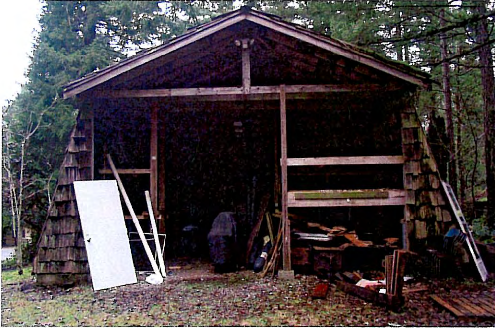
5. Front view of Maintenance / Wood Storage building.
