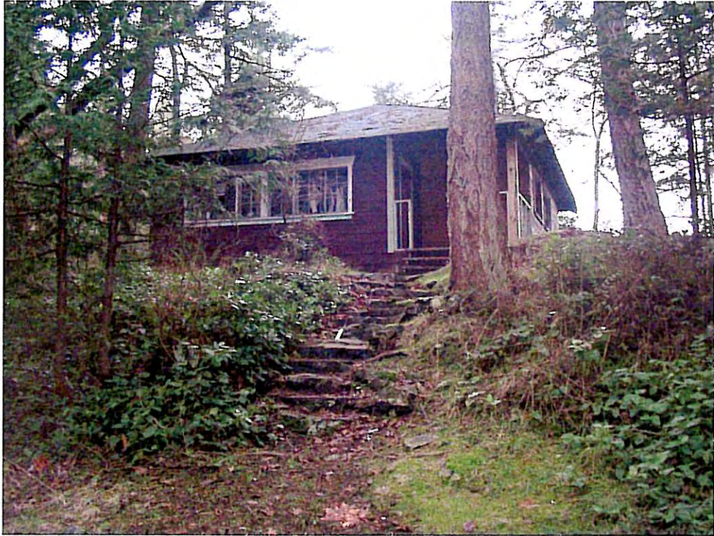
9. West entrance to abandoned Craft Hut building.
