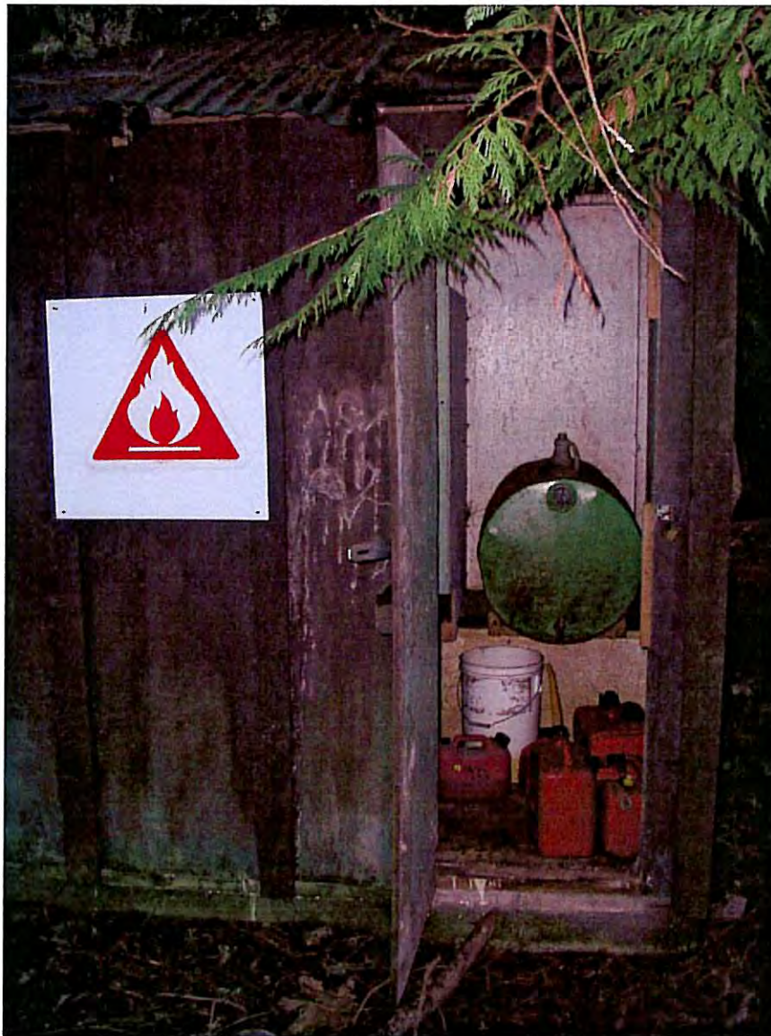
Figure 4. No large areas of stained soil or distressed vegetation were seen around the flammable liquids storage shed, located between Splash 1 and Cabin 2.
