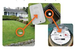
Reading your water meter: Look at the meter face. Is the leak detector (usually a black triangle or red star) moving? If so, and all sources of water in the house have been shut off, you have a leak.
