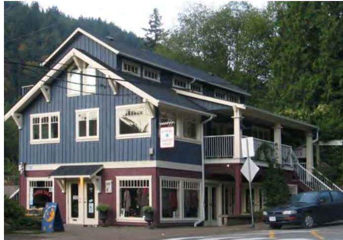
Example of third floor space built into the roofscape.
