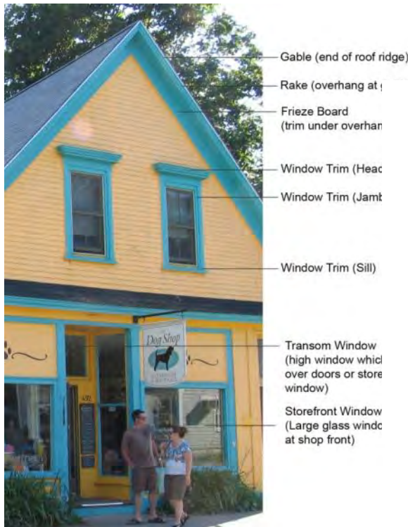
Illustration showing the use of frieze boards and other trim
