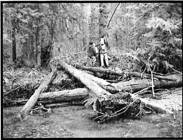
Centre Creek: Large Woody Debris Placement
