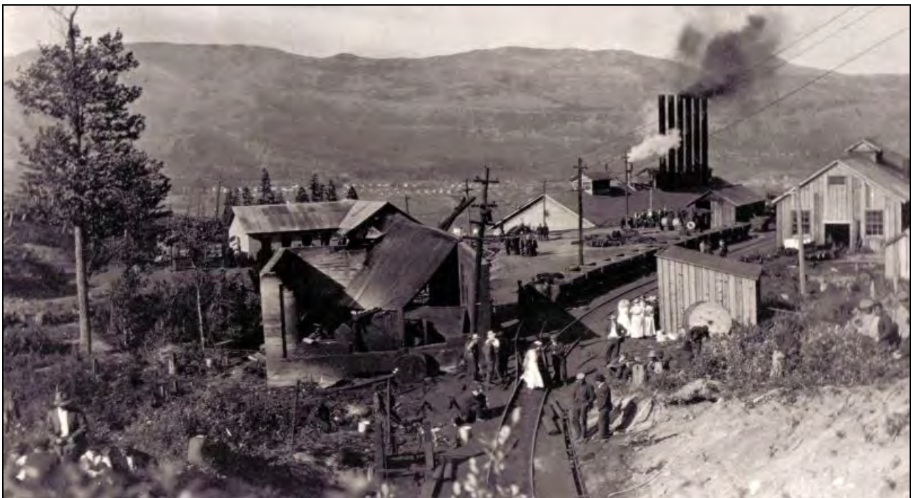
Engine house outside the No. 1 Mine entrance with the roof blown off and the concrete wall demolished by the explosion.
