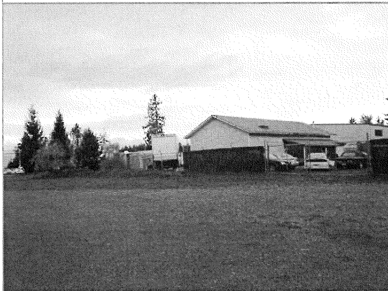
Picture 2: Auto sales area looking south east towards Alberni Highway, showing the auto sales office & garage from the rear.
