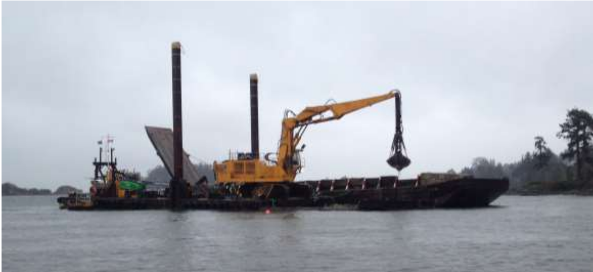
Photo: Dredging/blasting for the marine outfall during the winter fisheries window
