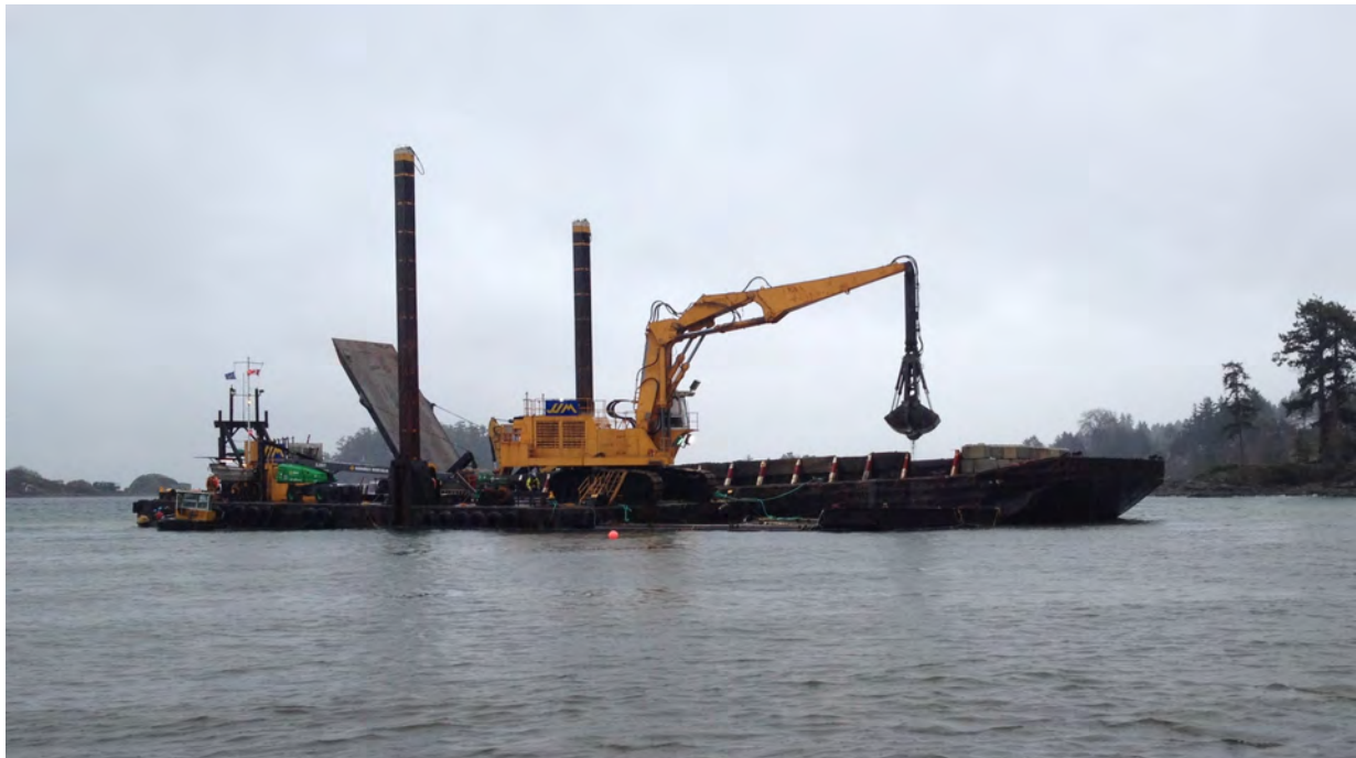
Photo: Outfall Construction Barge in Hammond Bay, January 2016.
