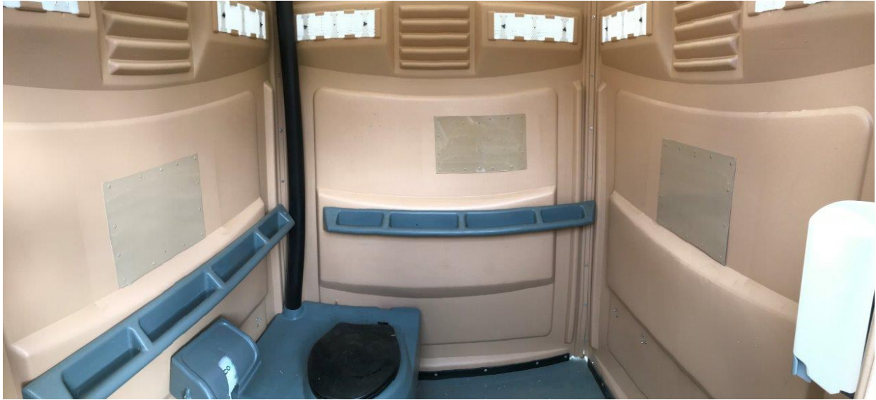
Repair to the unit by Parks Operations Staff
