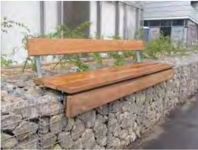
Figure 3a. Gabion Seat Wall precedent images.
