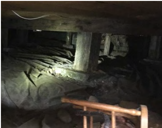
View in crawl space
