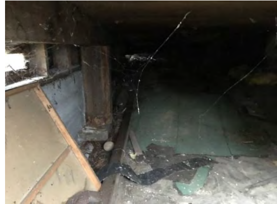
View in crawl space
