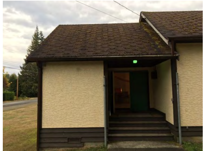
View of roof over entry
