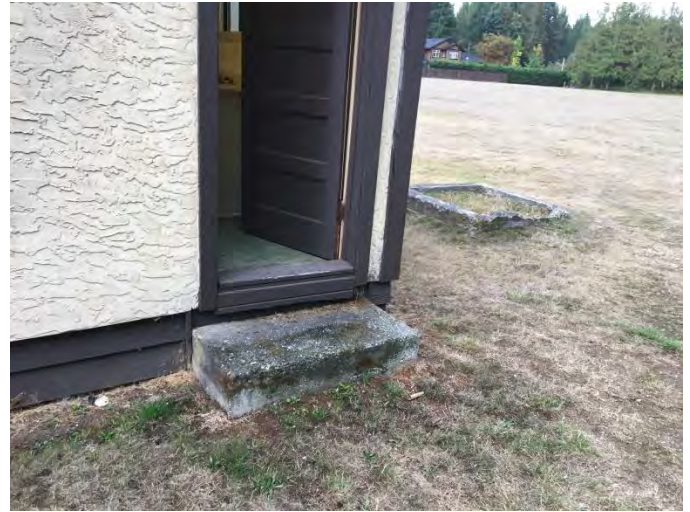
View of rear kitchen door
