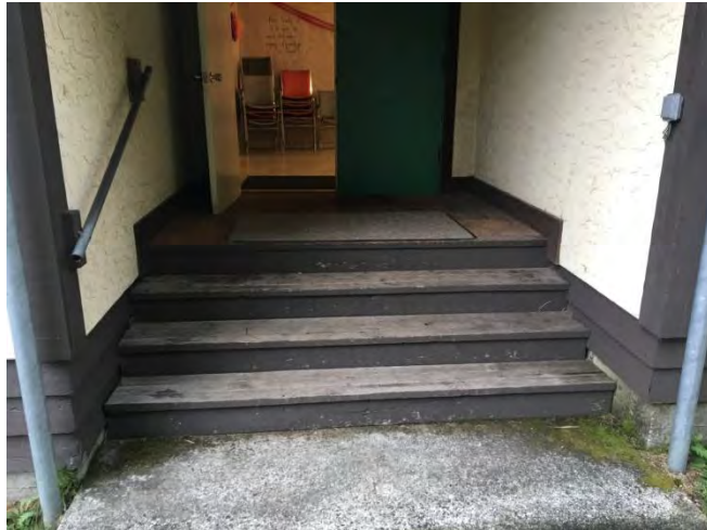
View of main entry door and stair
