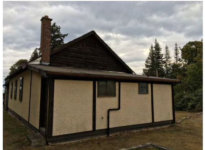
View of roof over rear of Hall
