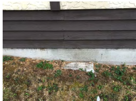
View of foundation
