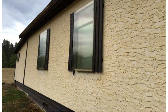
View of side windows
