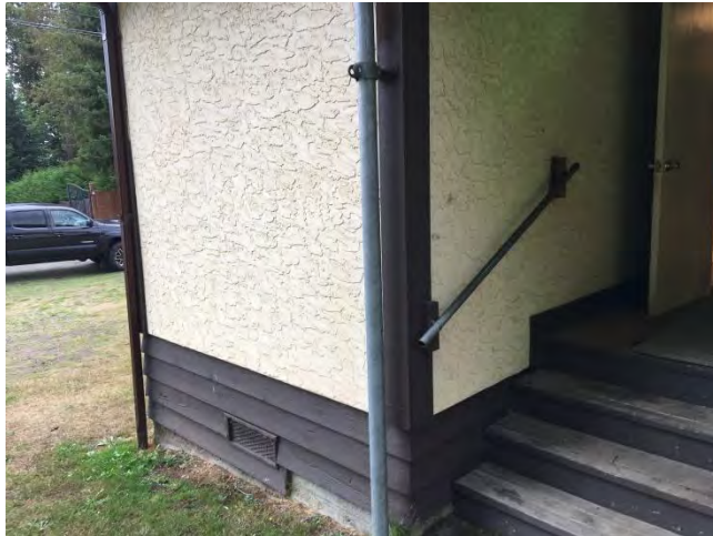
View of handrail at entry stair
