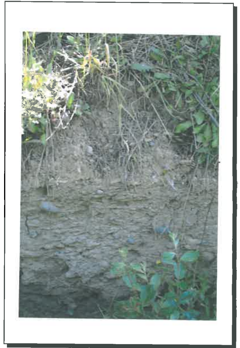
7b): Soil Pit #7, hard till profile in ditch at west P/L
