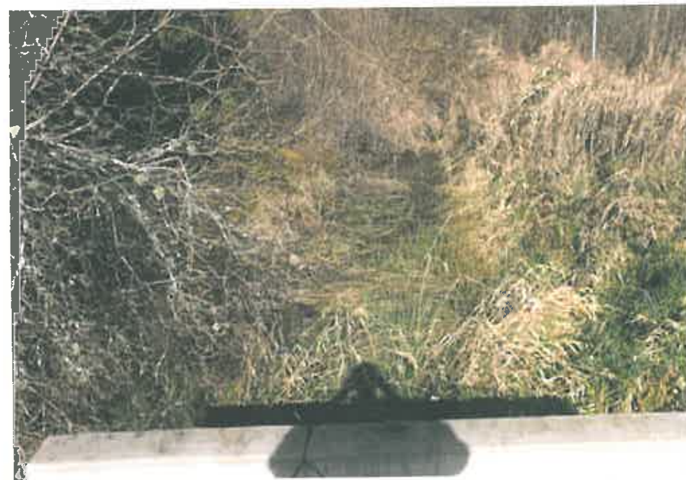
8(d): Ditch looking north at entrance
