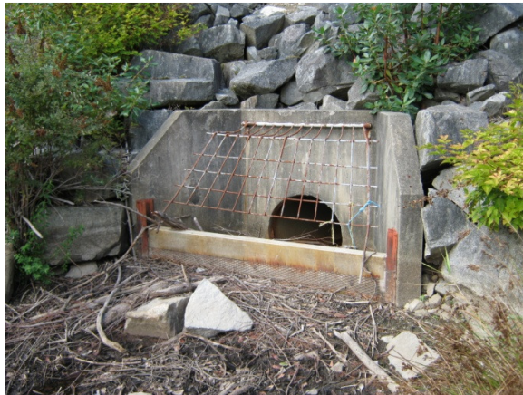
Enos Lake Outlet Structure
