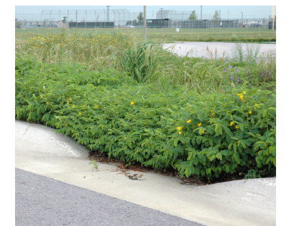
Curbs and curb cuts are addressed within the Standards in order to delineate road edge, ensure efficient access and direct stormwater run-off.
