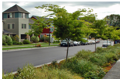
Raingardens adjacent the street absorb and filter stormwater while contributing to the streetscape aesthetic and pedestrian experience.
