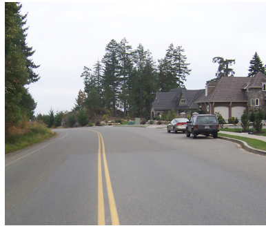
Fairwinds collector roads are overbuilt for the density of the community.
