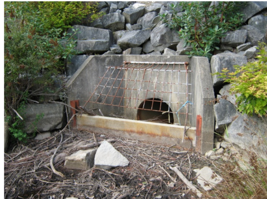
Enos Lake Outlet Structure
